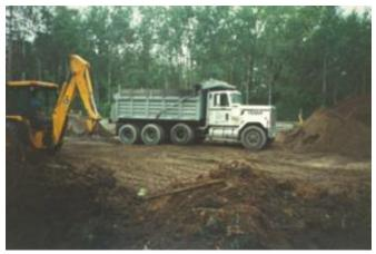
Treated over 500 tons of lead-affected soil from a former police pistol firing range with EnviroBlend and rendered soil nonhazardous. Placed treated soil on-site of the former firing range under the direction of the PaDEP under the new progressive Act II guidelines. Placed soil 20 feet below the parking lot of the new Home Depot constructed at the property, which saved transportation and disposal costs.
